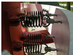
Figure 11. springs set (from Gerb)
